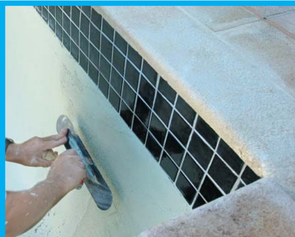
REGAL STONE IS TROWELLED ONTO THE CONCRETE SURFACE.
